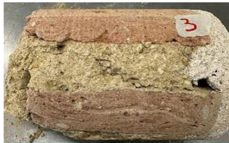
Renovation & reinforcement of old mortars
