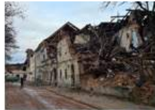
1. Collapsed URM buildings
