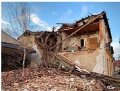
Collapsed unreinforced masonry building on Sremskaya St. in Petrinja. Photo by Denis Lazarević
