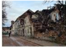
1. Collapsed URM buildings
